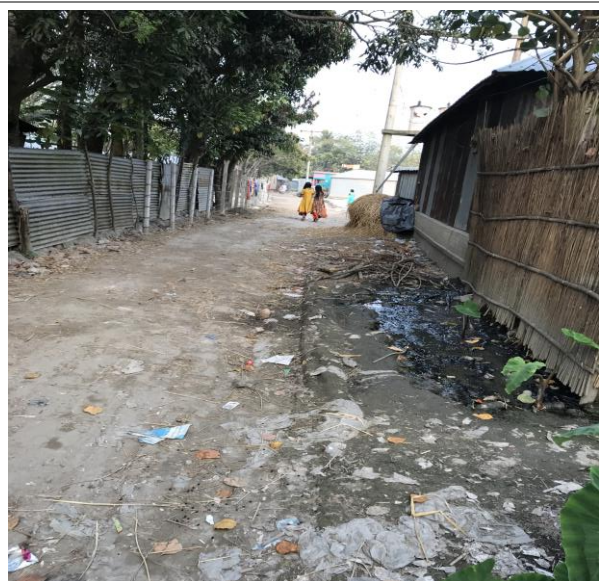
WARD-7 : (R4) RCC Road at Bhobanipur Azher-Afser Road to Shalghor via Apur's House, 720 m
