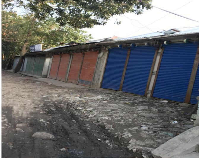
WARD-3 (R-8) CONSTRUCTION OF RCC ROAD GAGRAKHALI BERA MADHUPUR ROAD MOTIN SHOPS TOWARDS FIELD, LENGTH: 1190 M
