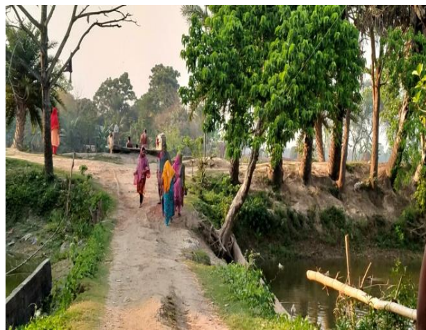
Ward-3: R-3: Construction of BC road at Gagrakhali Kashed House to Isamoti river Dayke Via laxmipur
