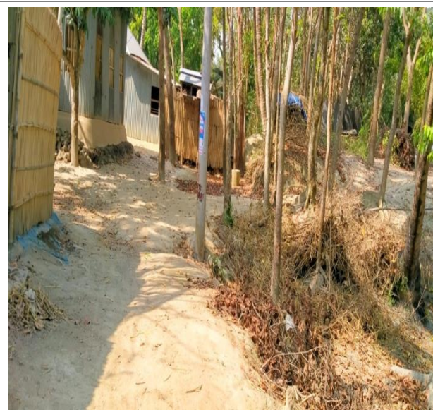
Ward-7: R4: RCC Road at Bhobanipur Azher-Afser Road to Shalghor road via Apu's house- Length-720 m
